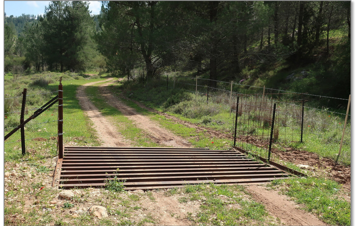
A cattle grid providing a secure boundary.
